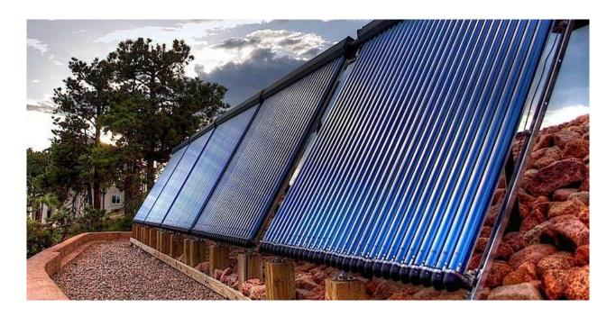
It is difficult to say which type of collector design is better. Each of them has both advantages and disadvantages: flat collectors are cheaper than vacuum ones;
